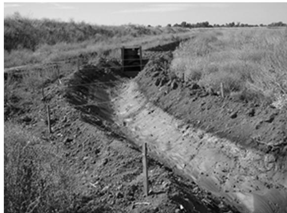
*recently installed sediment trap in Yolo County*
